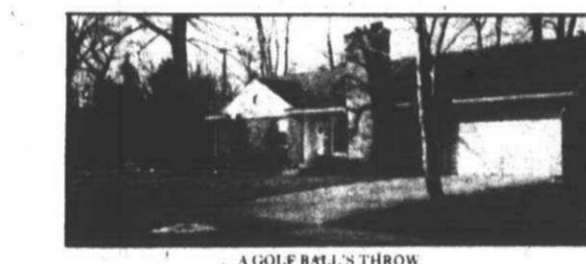
A GOLF BALL'S THROW To Western Golf & Country Club. This 3 bedroom custom built broadfront ranch is nestled peacefully under towering trees on almost 1/2 acre lot in Redford's most distinctive area. Offers central air conditioning, spacious kitchen, formal dining room and family room. Land contract terms or 9 1/2% conventional mortgage. Move in condition at $45,900. S 041 Call Vince Vornhagen 477-6300 or 522-1258 WESTDALE CO.
