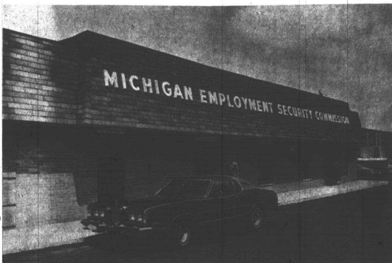
THE NEW Michigan Employment Security Commission building on Joy Road, between Haggerty and Lilley roads in Plymouth Township, is now open for business. The building replaces the former MESC office located on Mill Street. (Staff photo by Maurie Walker)
