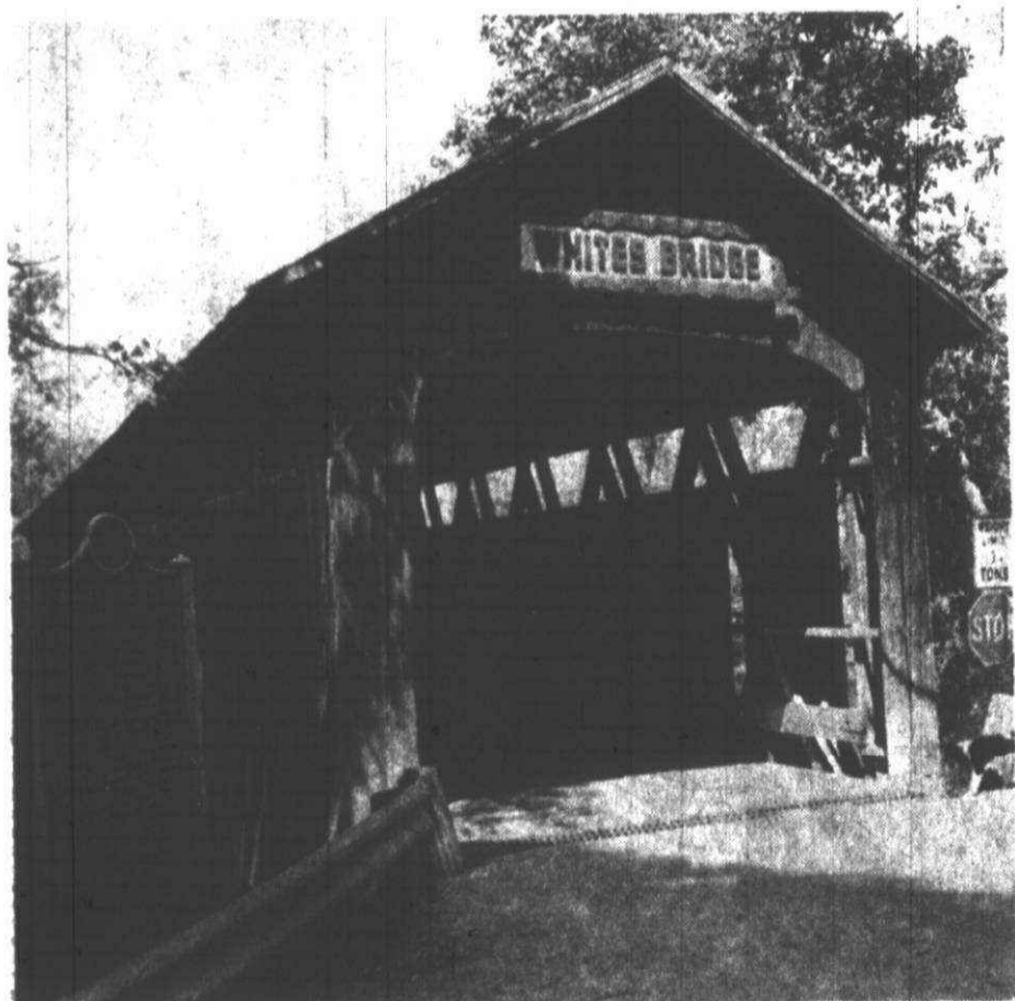
WHITE'S BRIDGE near Belding.
