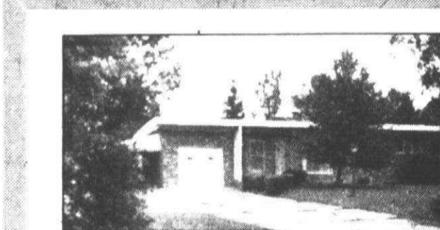
LIVONIA Brick ranch with attached garage plus a large carport. Partially finished basement, 2 fireplaces, 2 full baths, 1st floor laundry room. Approximately 2/3 acres of country living located in a super area. $49,900 Call 261-0700 (49813)
