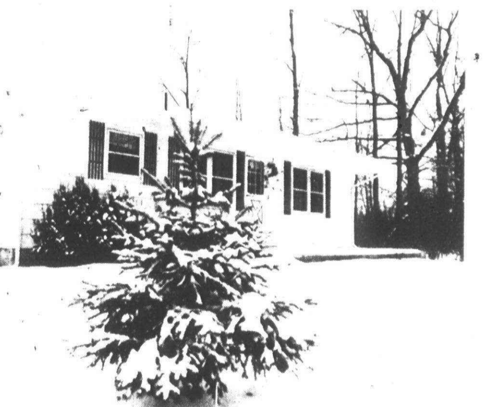
Len Mason, of 4533 Corrine, Canton, is quite proud of this home he built from the ground up and isn't overjoyed about the news that the township may condemn the neighborhood for an industrial park and relocate him with federal grant money. (Staff photo by Gary Caskey)
