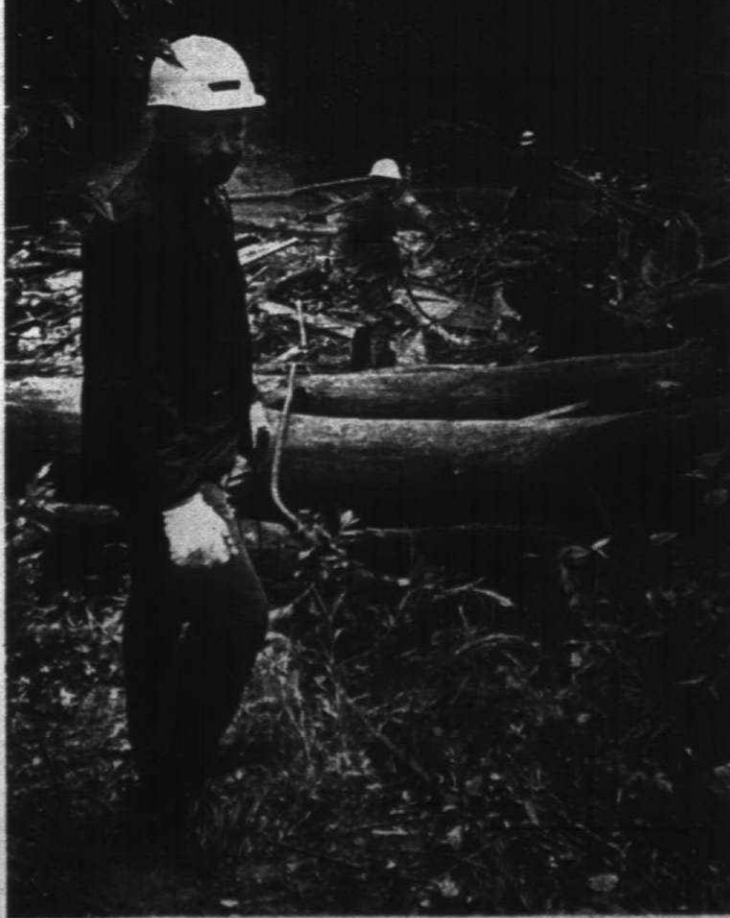
Larry Jacobs of the Wayne County Parks and Recreation Dept. supervises cleanup of a log jam at last year's cleanup. Clearing logs and fallen trees increases the river's flow and is an important factor in easing pollution, according to experts.
