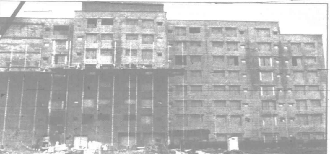
Construction of a low-income senior and handicap housing project on Sheldon and Ford roads is expected to be complete by September.
