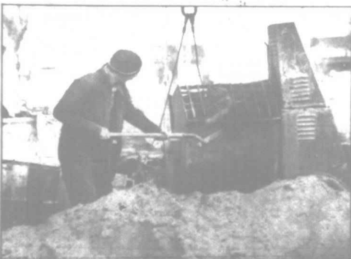
A construction worker mixes mortar for brick work.
