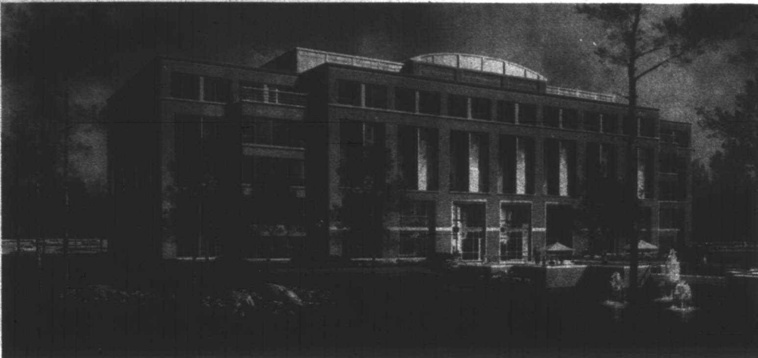
Victor V will have a two-story lobby, locker and shower facilities, surface parking for approximately 480 plus reserved executive parking.
