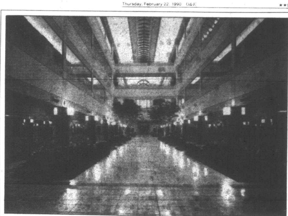
Award winner Laurel Park Place, Livonia, has been named one of the winners of the Construction Association of Michigan award for the office and parking structure portion of the development. R.E. Dailey of Southfield was the contractor.
