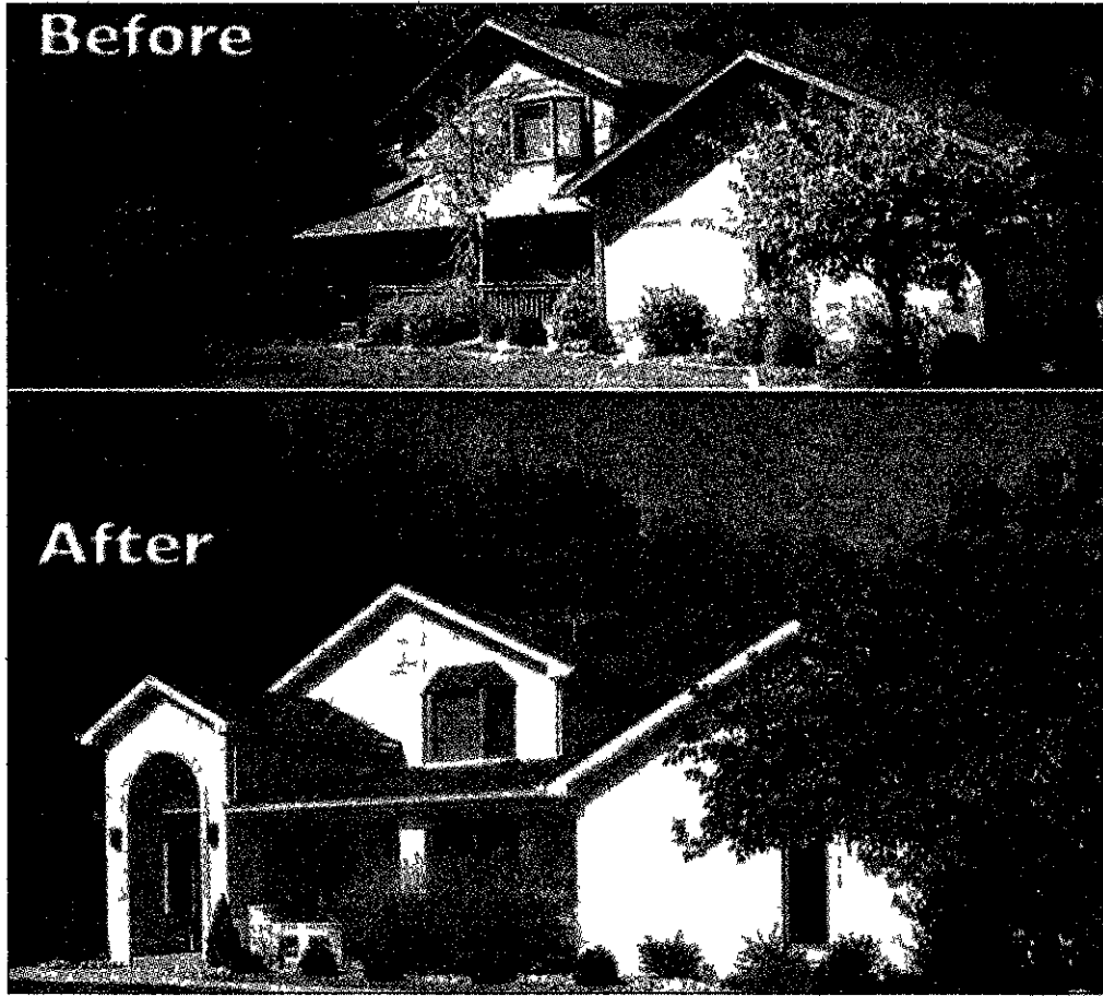
A remodeling system that achieves stonelike finishes has also been shown to reduce heating and cooling costs.
