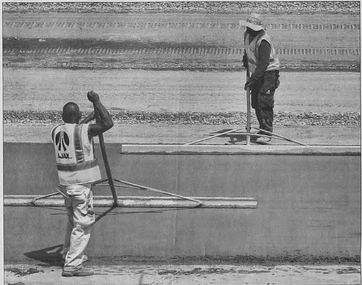
Some hand-finishing is required before the concrete sets.
