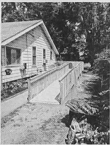
A wheelchair-bound mother and her daughter, who uses a walker, will have an easier time getting around their Farmington Hills home, after Safe at Home replaced steps with a ramp.
