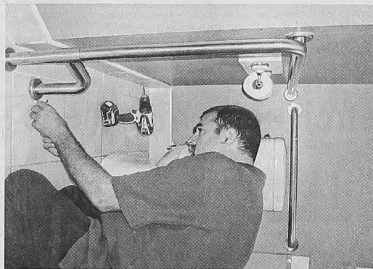
Tom Reuter, an employee of Evangelical Homes of Michigan, installs a grab bar in a bathroom, making the home safer for its residents.
