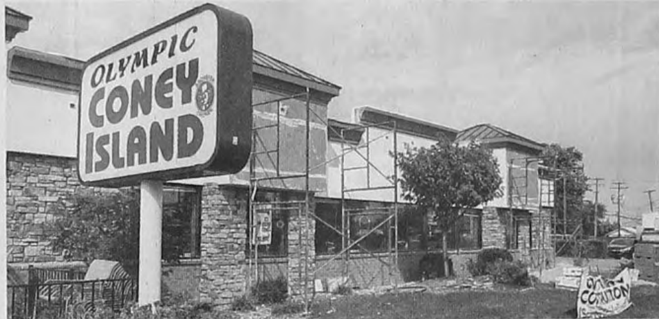
New stone and stucco, along with a new roof, are the visible renovations for Olympic Coney Island in Westland.
