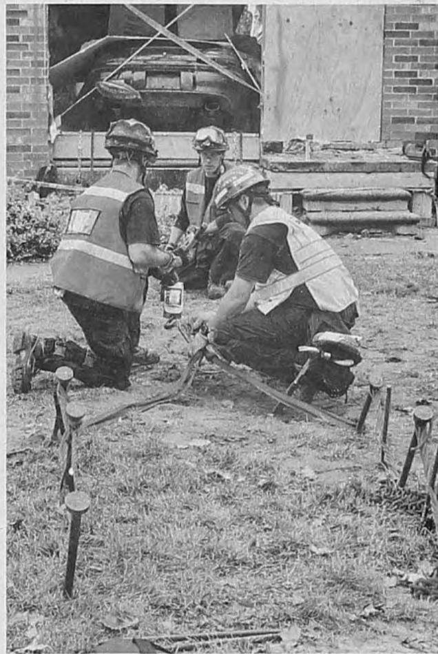
The car is stabilized with a chain that leads outside to a series of stakes driven deep into the ground.
