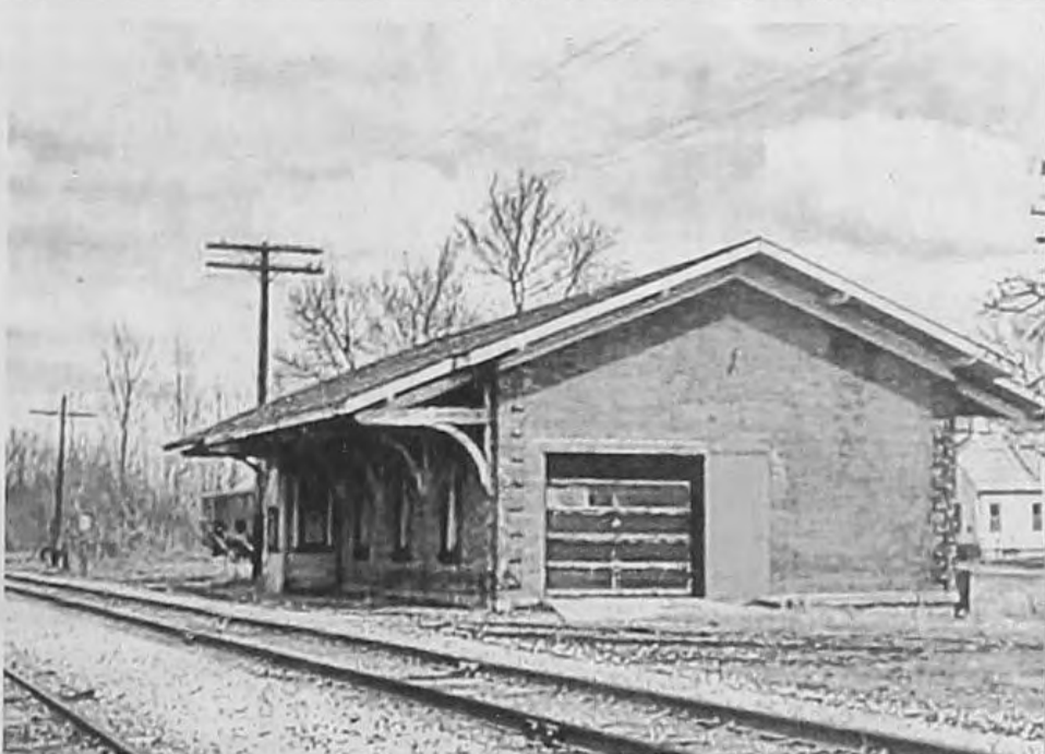
The since-restored 1859 Grand Trunk RR Depot in New Haven, Shiawassee County.
