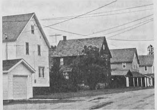
Company-built 1910 homes in Fulton, Keweenaw County.
