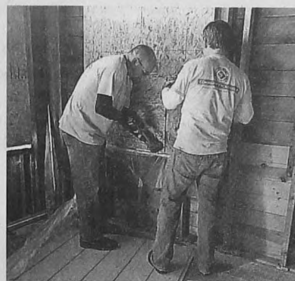
Work continues on the Village Arts Factory site.
