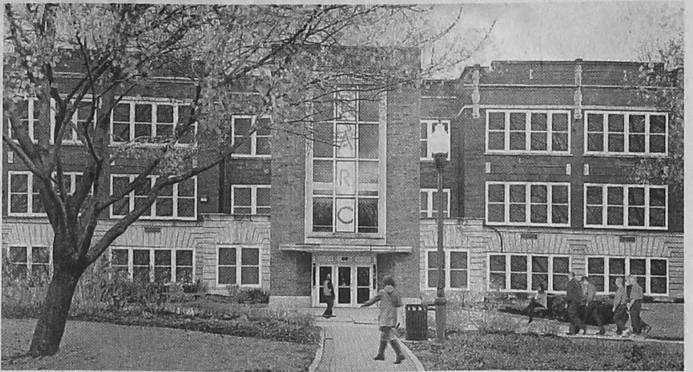
With all new windows, this is how the front of PARC would look after a massive renovation project. PARC
