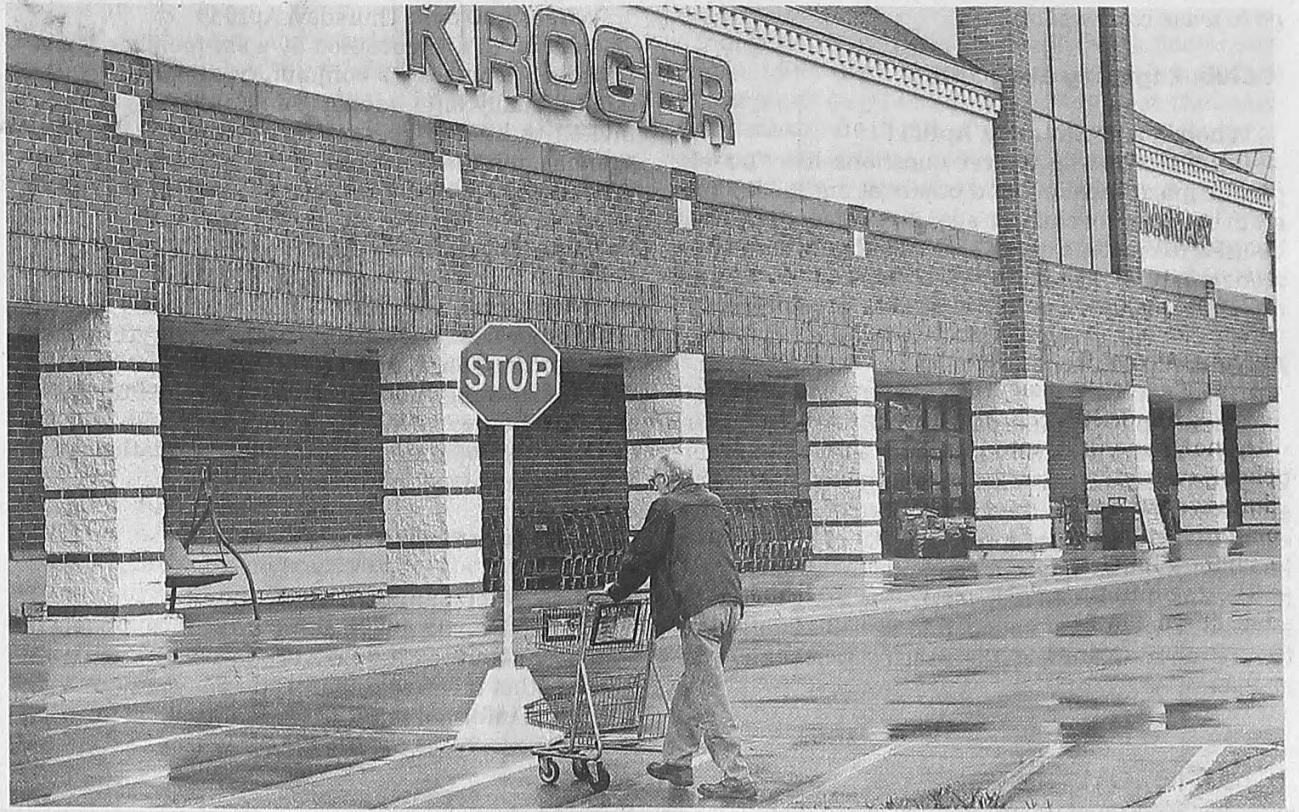
The Kroger store on Haggerty Road in Northville Township has received a $3.5 million makeover. BILL BRESLER | HOMETOWNLIFE.COM
