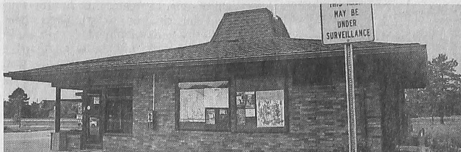
The building containing restrooms at the rest area along I-275 in Canton. The Michigan Department of Transportation recently announced the rest area would close in November. DAVID VESELENAK | HOMETOWNLIFE.COM
