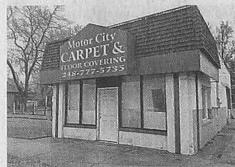
The proposed brewery will open in the former Motor City Carpet store at 27719 Seven Mile Road in Livonia.
