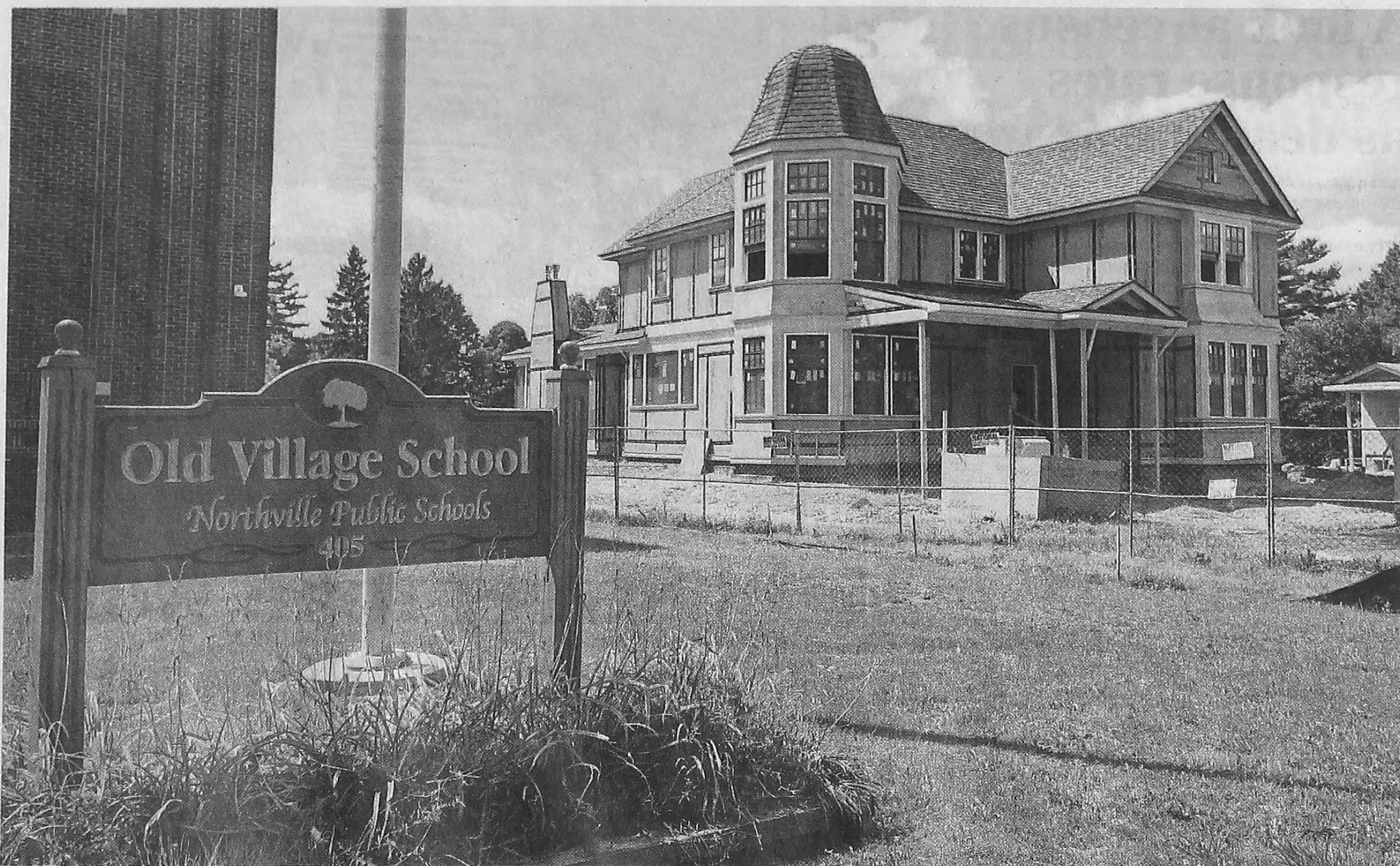
Three homes are being built along West Main Street in Northville on the property of the former Main Street School. PHOTOS BY JOHN HEIDER/HOMETOWNLIFE.COM
