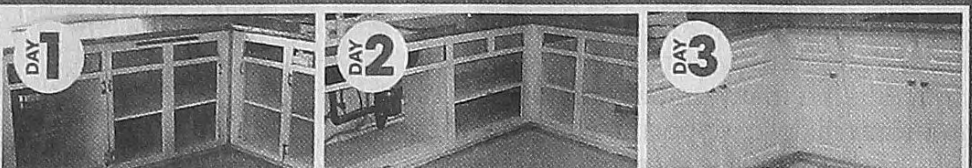
DAY 1 Existing cabinets are prepared for the refacing process
